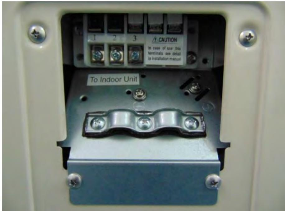
Picture No.5 : Terminal of outdoor unit model: RAS-10PAVPG-E
