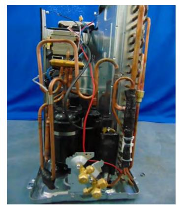
Picture No.6: Compressor compartment of outdoor unit model: RAS-10PAVPG-E
