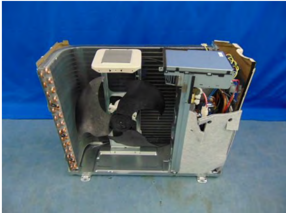
Picture No.3 : Inner view of outdoor unit model: RAS-16PAVPG-E
