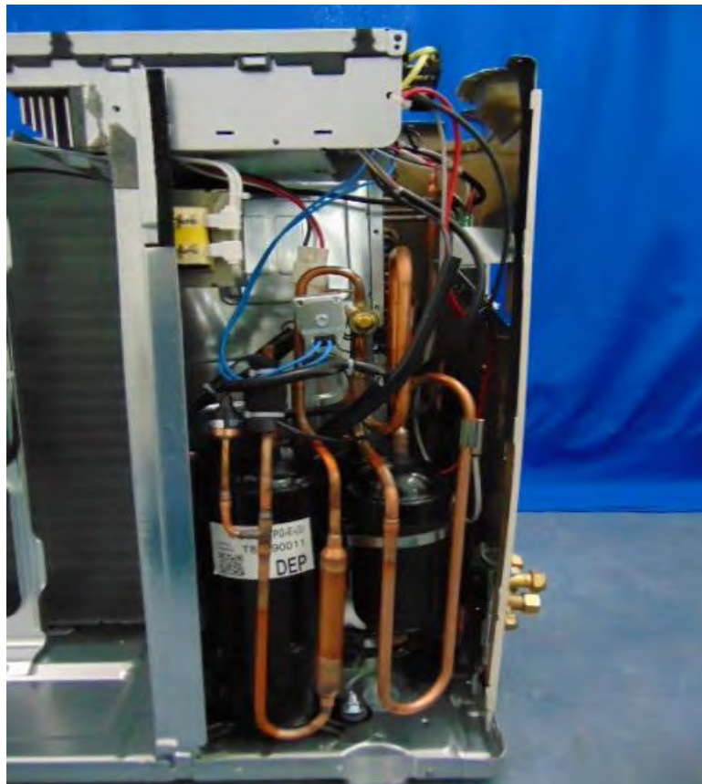
Picture No.6 : Compressor compartment of outdoor unit model: RAS-16PAVPG-E
