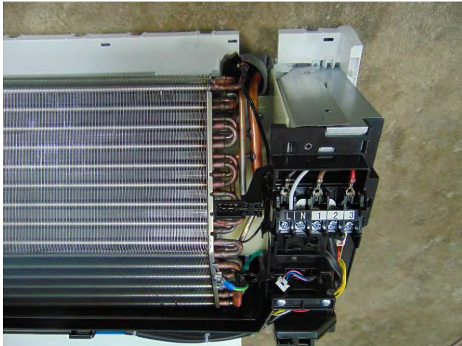
Picture No.46: Terminal view of indoor unit model: RAS-B16J2KVRG-E
