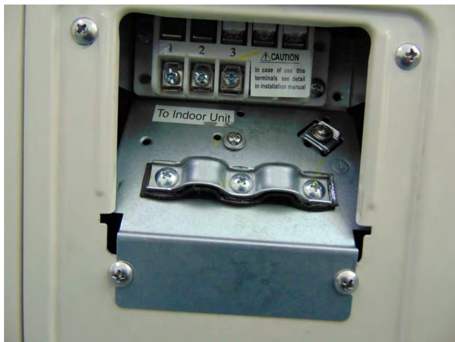
Picture No.20: Terminal of outdoor unit model: RAS-22J2AVRG-E
