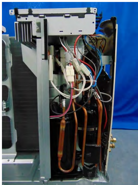
Picture No. 26: Inner side view of outdoor unit model: RAS-24J2AVRG-E
