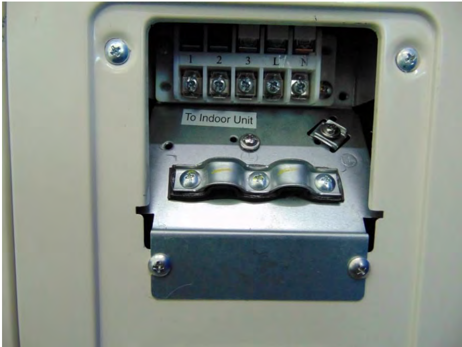
Picture No.27: Terminal of outdoor unit model: RAS-24J2AVRG-E
