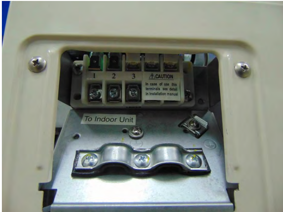
Picture No.13: Terminal of outdoor unit model: RAS-16J2AVRG-E
