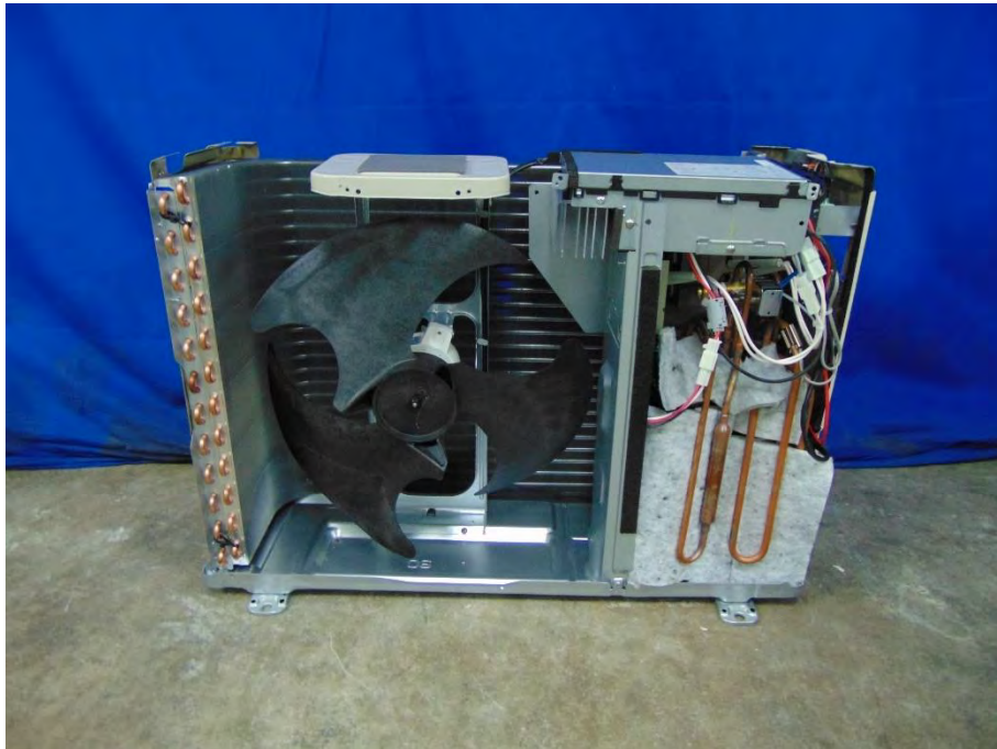
Picture No.23: Inner view of outdoor unit model: RAS-24TAVG-E
