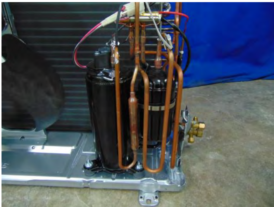
Picture No.26: Compressor compartment of outdoor unit model: RAS-24TAVG-E
