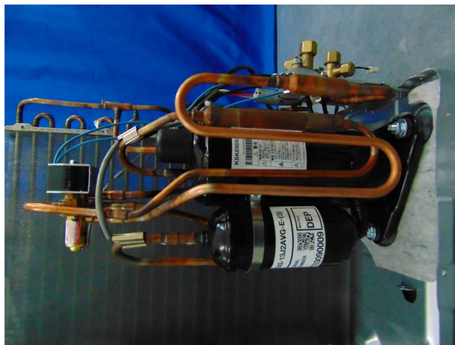
Picture No.12: Compressor compartment of outdoor unit model: RAS-13TAVG-E
